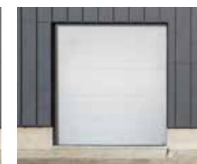
REPAIRED DOOR WITH AMARR 2747 REPLACEMENT SECTION
